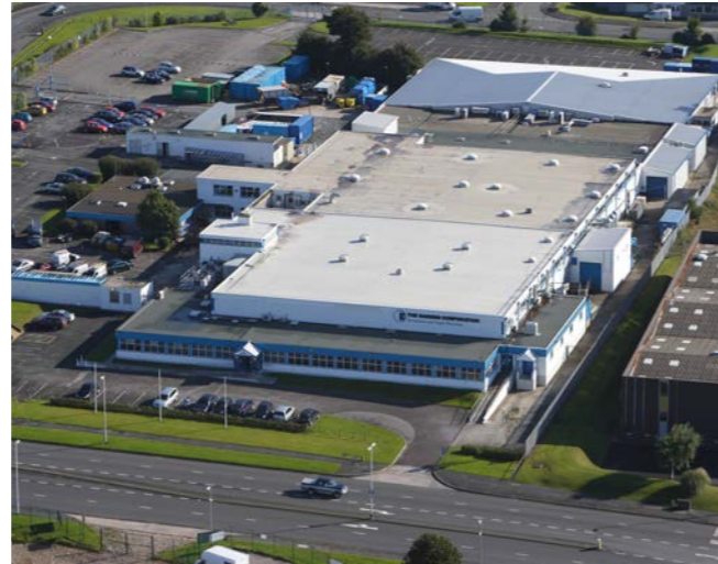
Barden UK plant, Plymouth, United Kingdom
