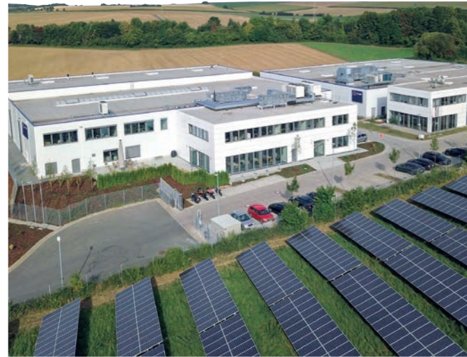
HQW Precision plant, Kürnach, Germany
